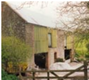
72 - Lincombe Barn, Lincombe
