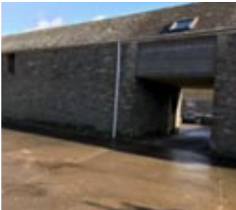
81 - Houghton Farmhouse and Barns, Houghton
