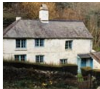
54 - Foxhole Cottage, Foxhole
