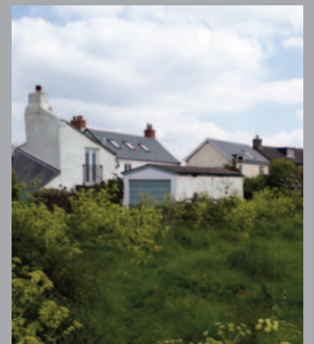
• LARGE CHIMNEY BREASTS ARE VISIBLE
