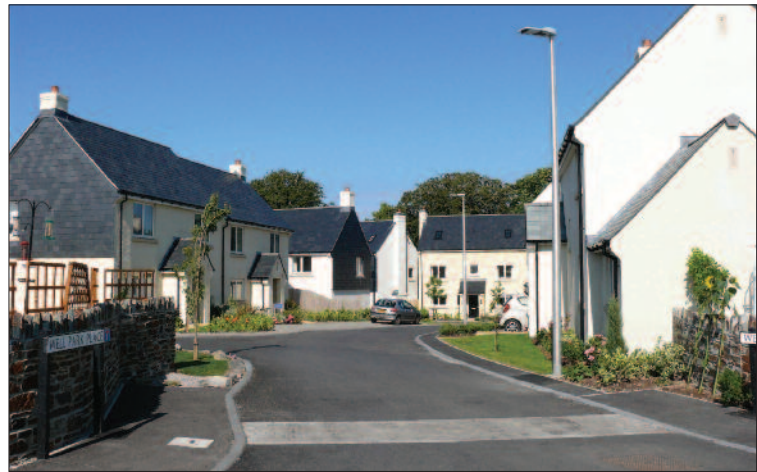
New houses in School Road
