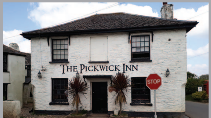
EXAMPLES OF LISTED BUILDINGS
