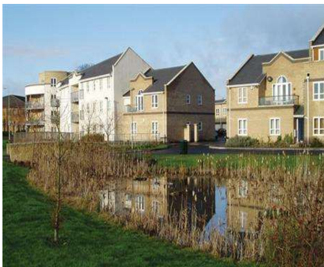
Sustainable Drainage, Attenuation pond housing scheme, Oxfordshire © Environment Agency
