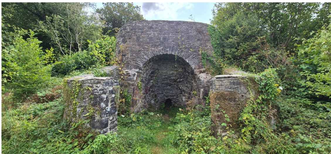
FIGURE 21: EXAMPLE OF A COMPLETE LIME KILN AT HOYLE COPSE
