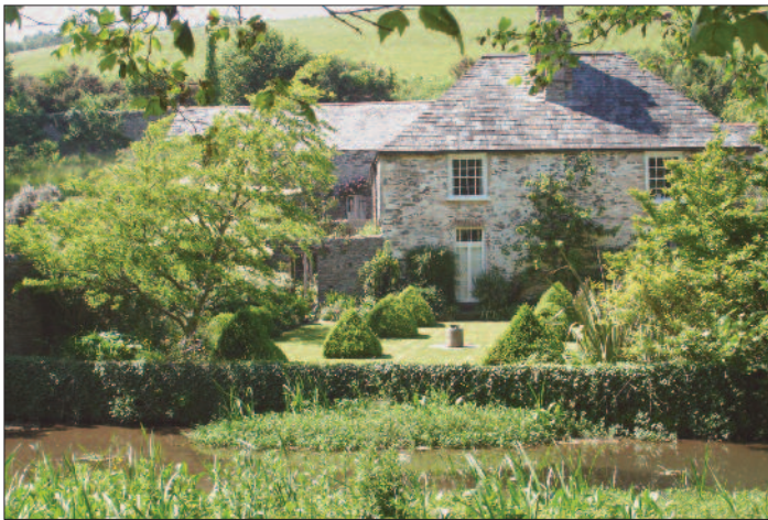
Riversbridge - a listed building
