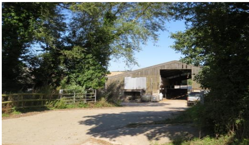
Photograph 7.2 Access road to The Dairy site from Milton Lane
