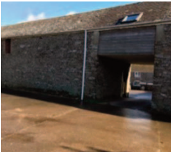
81 - Houghton Farmhouse and Barns, Houghton
