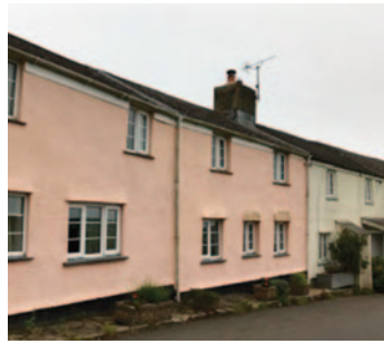
2 - 1 and 2 Court Cottages, Bigbury Village
