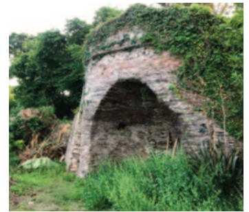
67 - Lime Kiln, Milburn Orchard, Stakes Hill
