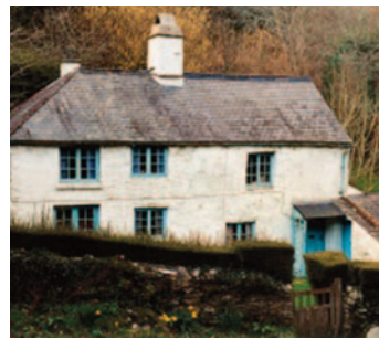
54 - Foxhole Cottage, Foxhole
