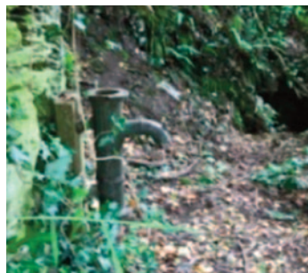
17 - Water Pump, Cot Lane, Lower Bigbury
